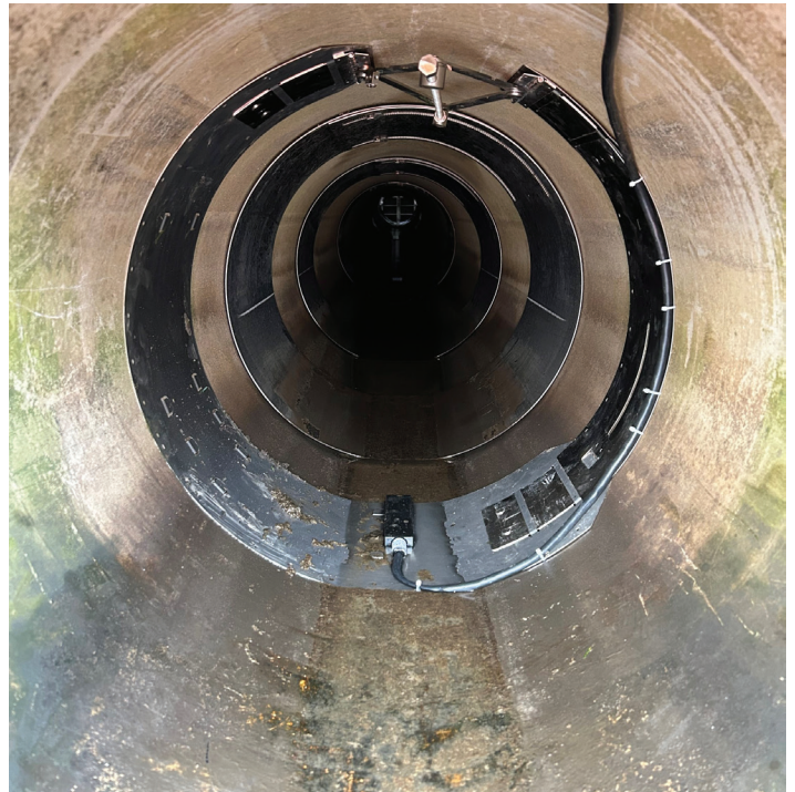
Teledyne ISCO's TIENet 350 Ex area velocity sensor installed in a discharge channel.
